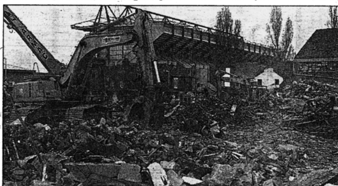
RUBBLE: The site of the demolished Liberty Building
